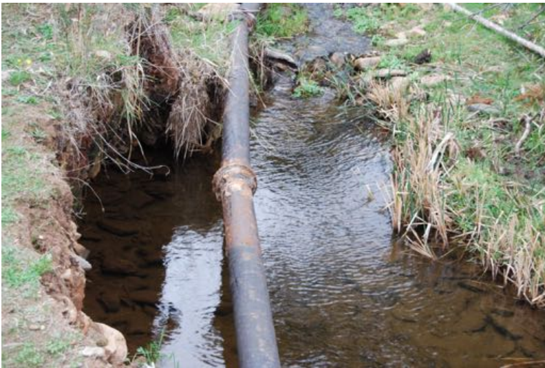
^Andrew explains about the Mitcham works piping qExposed old cast iron piping
